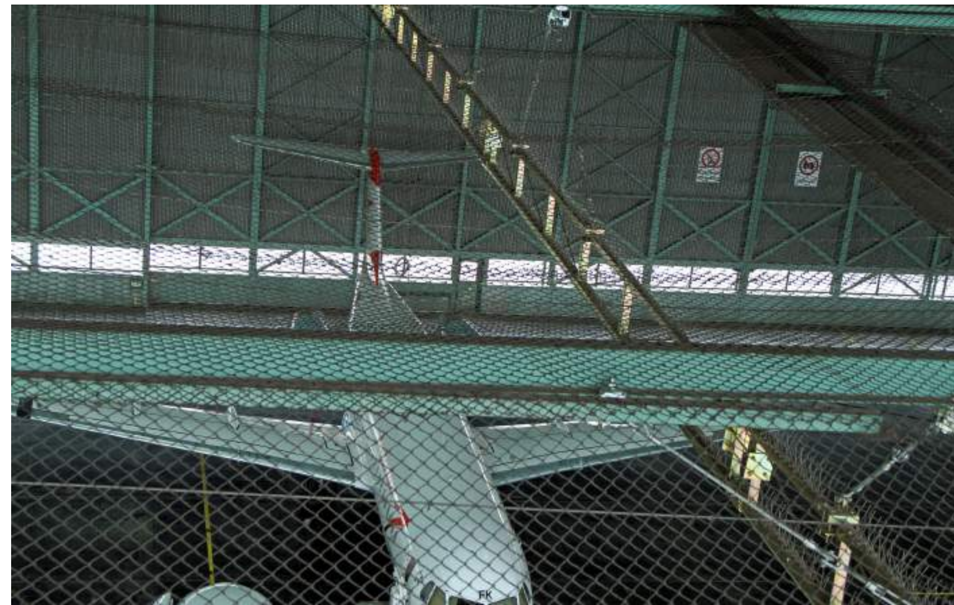
Ceiling mounted track system positioned above the aircraft to provide workers access to the full length of the airplane.
