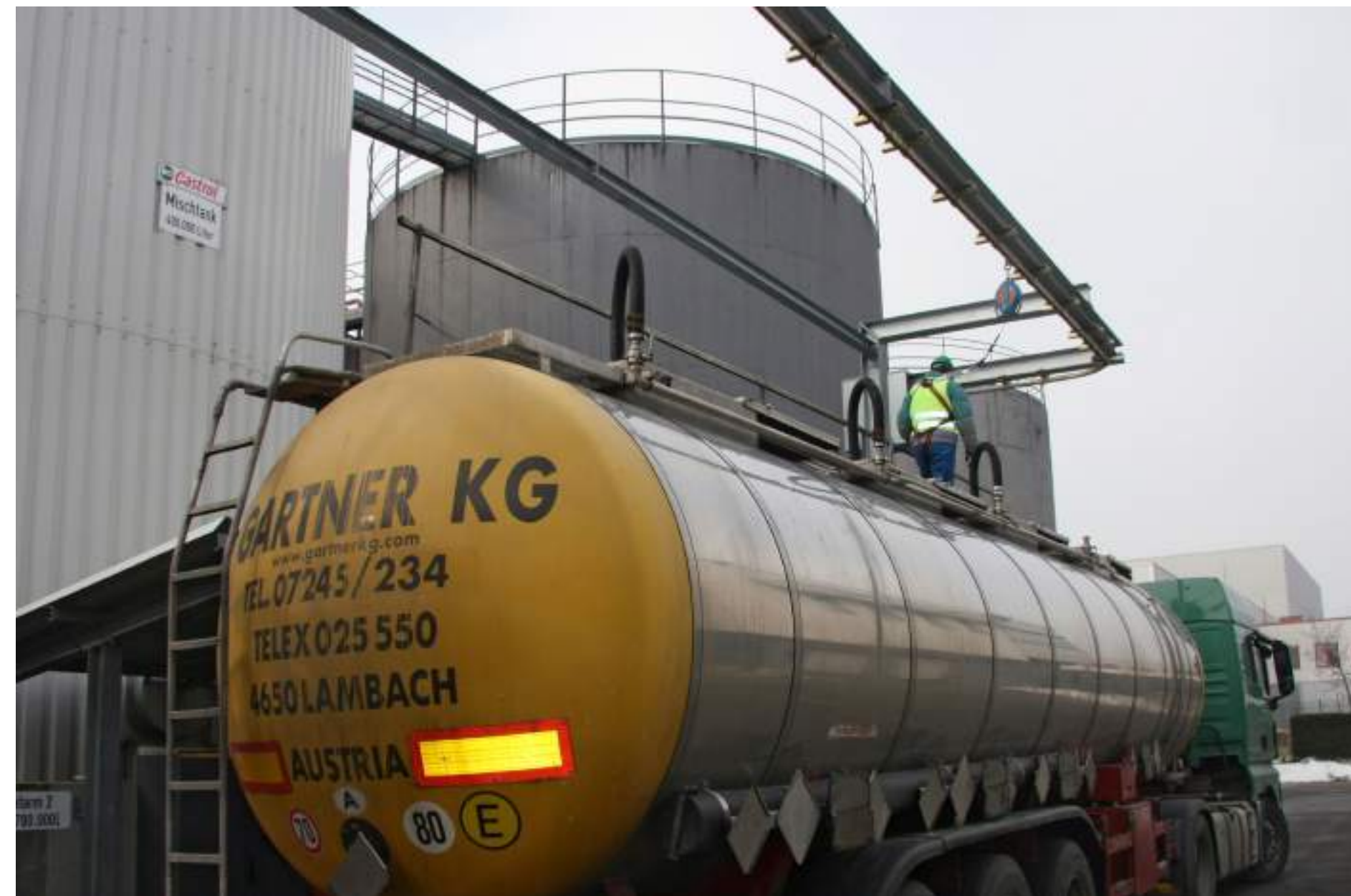
Freestanding fall arrest track bend system for outdoor service processes in trucks.
